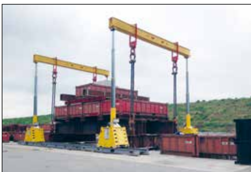
◀ SL-400 Gantry during load testing.
